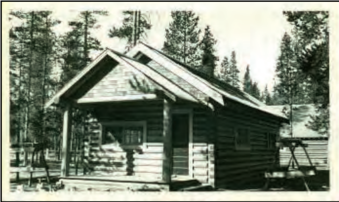
The historic Madison Ranger Station office building was constructed in West Yellowstone, Montana, in the 1920s.
