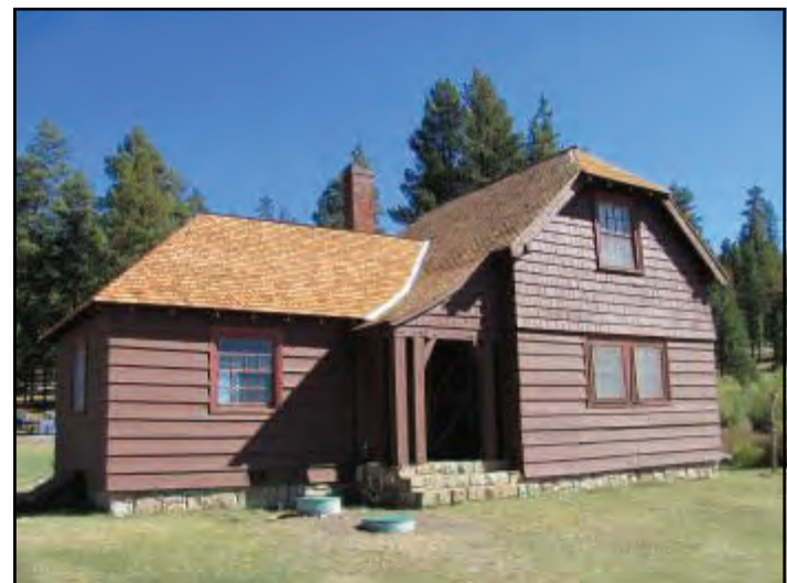
ARRA funding restored the 1930s Allison Ranger Station office, (above), warehouse, residences, and other structures for use.
