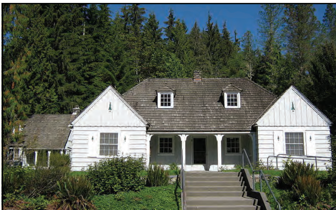
Verlot Public Service Center as it appears today.
