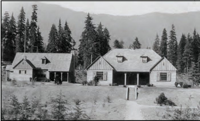
Historic Monte Cristo Ranger Station in June 1938, with the protection assistant's residence on the left. U.S. Forest Service photograph courtesy of Darrington Ranger District
