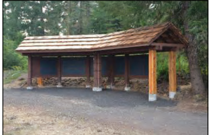
The newly-constructed but yet-to-be finished Fish Lake Historic Area kiosk as it appeared in September 2011.
