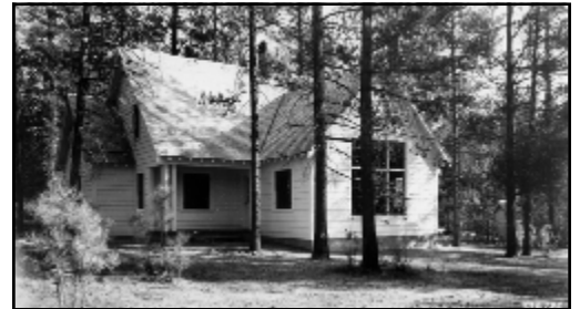
The crew house, built in 1935, was later used as the administrative building and remains in use. Photo was taken in 1936.
