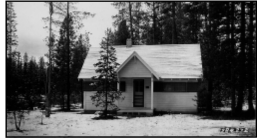
The headquarters building was constructed during the summer of 1931 for $450.
