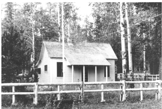
Gotchen Creek Ranger Station, Columbia National National Forest. In 1935
