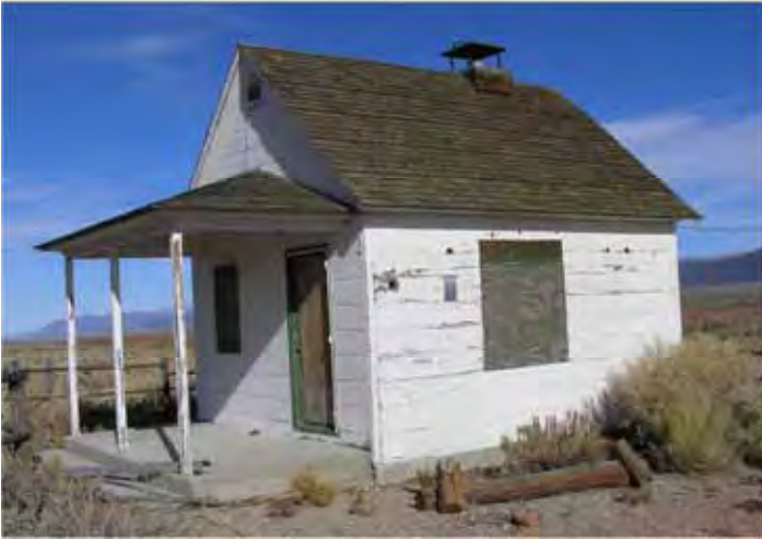
This 1933 structure is destined for the High Desert Museum. Photograph by District Ranger Steve Williams
