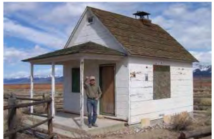
Reese River Ranger Station office building, Toiyabe National Forest, 40 miles south of Austin, Nevada, 1962-2008. Bob Boyd of the High Desert Museum on front porch in March 2008.
