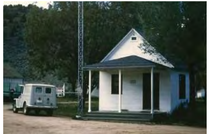
Bridgeport Ranger Station office building, Toiyabe National Forest, four miles northwest of Bridgeport, California, on U.S. Highway 395, 1933-1962.
