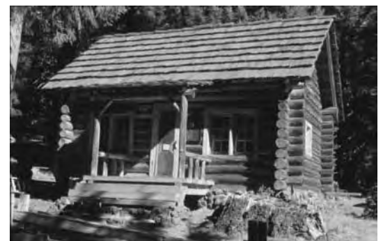
Dispatcher's office cabin after renovation in recent years replaced roof, porch.
