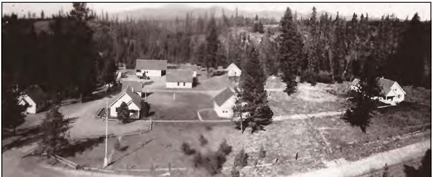
Blue Mountain Ranger Station, near Bates, Oregon. Buildings in foreground (left to right): CCC camp cookhouse, office, assistant ranger residence, and ranger residence. Warehouse, shops, garage, ice house, etc., are in background. Barracks are in the trees.
